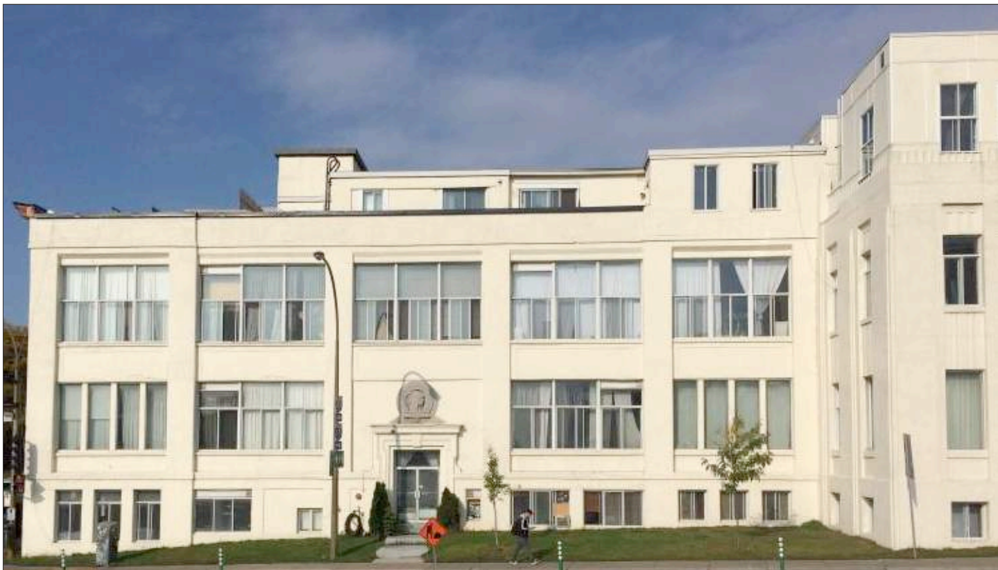
The ASN Building at the corner of de Maisonneuve and Décarie.
